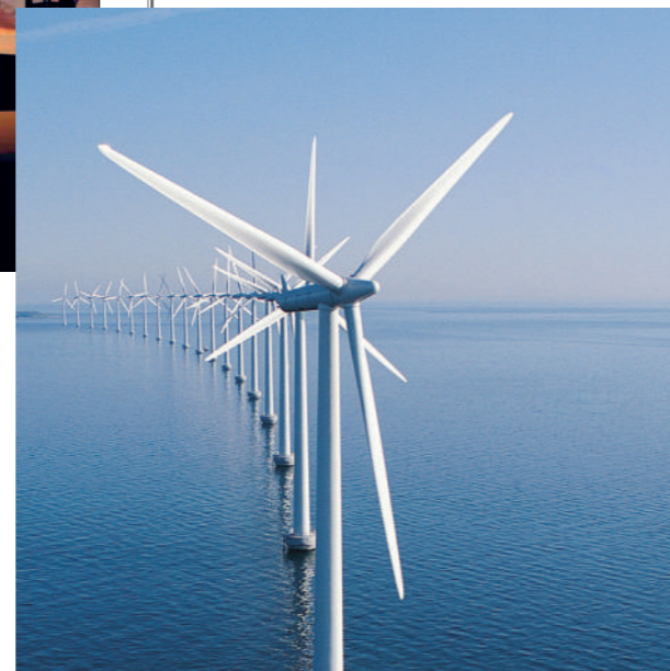
Wind driven generator
